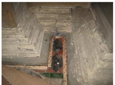
The floor under the carpet and the underlay is glazed tiles. There was considerable dampness on the surface of the tiles and it was noticeably greater at the margin adjacent to the base of the tomb. Note the extent of the corrosion occurring on the metal component of the gripper rods.
