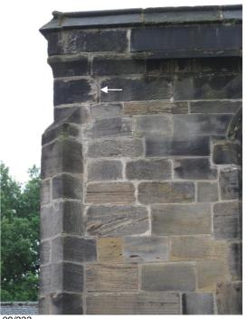
It appears that some relatively recent pointing has been carried out on this elevation but the upper east section has either subsequently moved or was not properly repaired as there are open joints as indicated by the white arrows.
